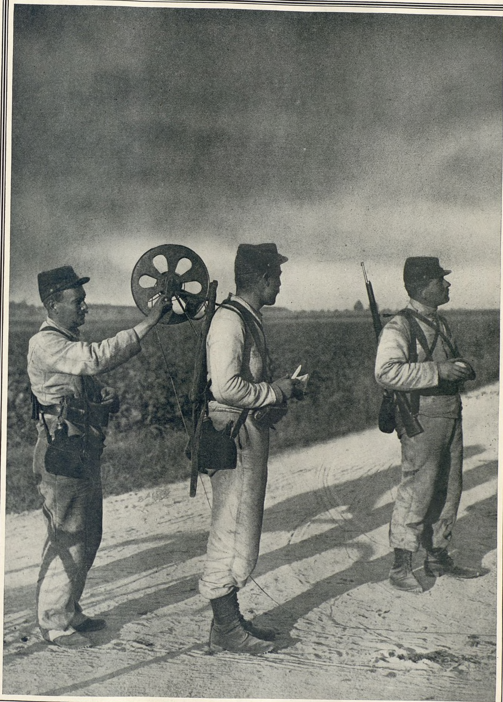
A TELEGRAPH DETACHMENT OF THE FRENCH ENGINEERS REPAIRING TELEGRAPH LINES NEAR THE FRONT
