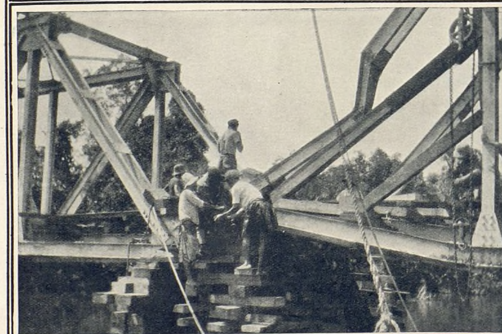
Repairing a Bridge Blown up by the Germans near Duala.—The Eastern Railway, along which the French troops are operating, starts from Duala; the Northern Railway, which was used in the advance to Baré, starts from Bonaberi. After the bombardment of Duala by H.M.S. "Challenger" the Germans evacuated the town along both these lines and made for other places, where vigorous stands were made against the advance of the Allies.
