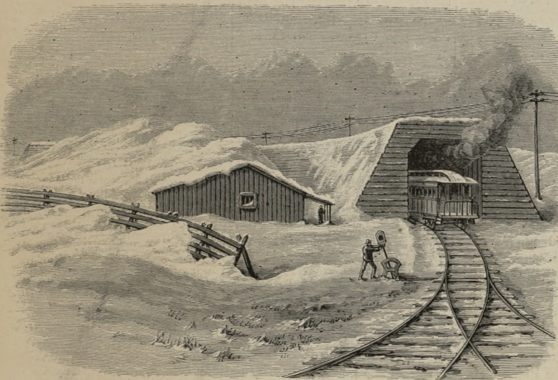
SNOW-SHED AND DRIFT-FENCE NEAR PIEDMONT.
