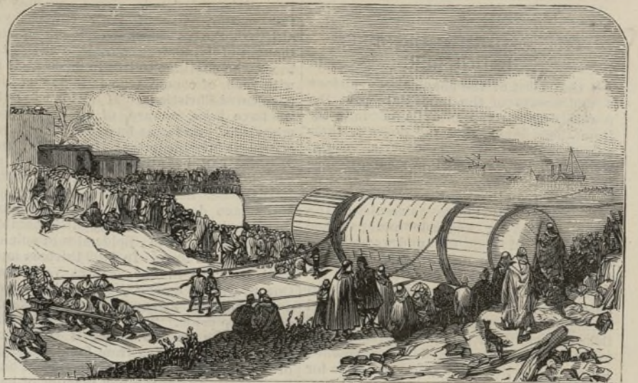
EGYPT.—LAUNCHING THE CAISSON CONTAINING CLEOPATRA'S NEEDLE, AT ALEXANDRIA
