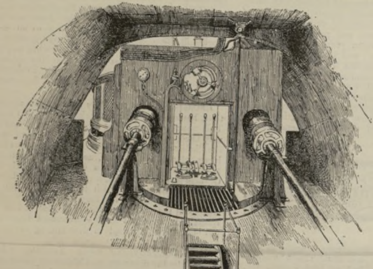
Cylinder containing Hydraulic Ram VIEW OF HYDRAULIC RAMMERS FOR LOADING GUNS, H.M.S. "RODNEY" The sketch also shows the upper part of the ammunition hoist casings and the levers by which the hoists and rammers are worked
