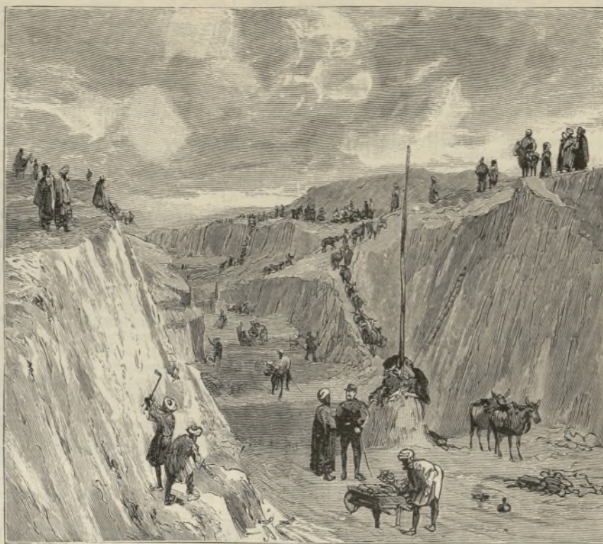
MAKING A CUTTING—ASSES TAKING AWAY THE EARTH IN PANNIERS
