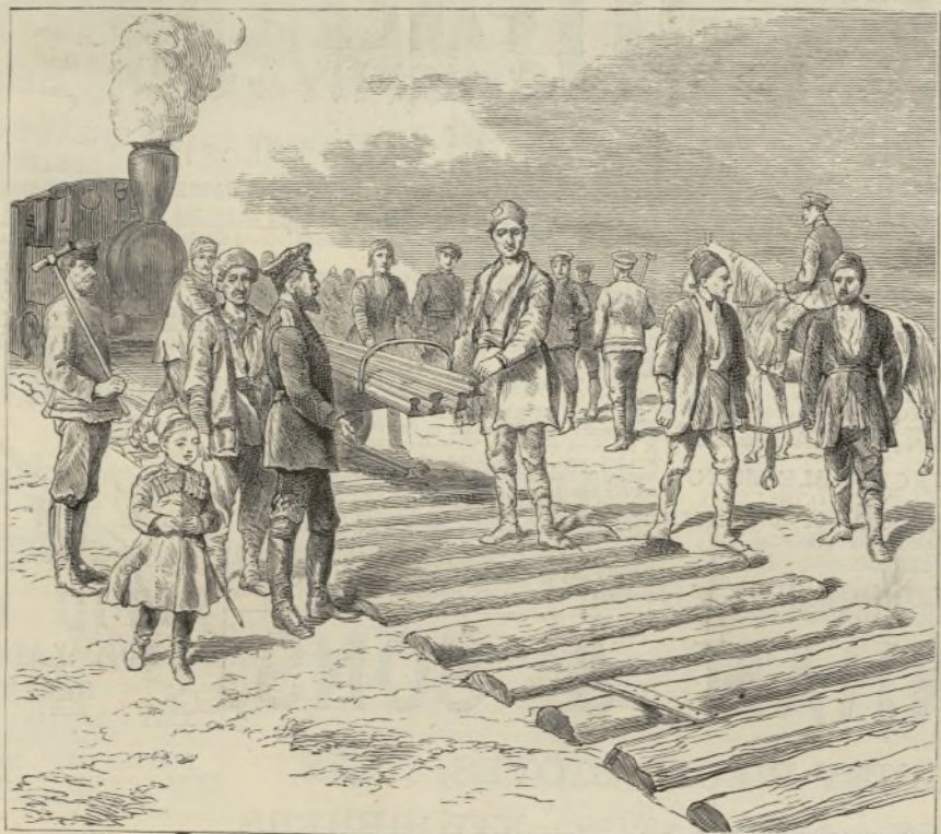
AT THE HEAD OF THE LINE—LAYING THE RAILS AT THE RATE OF FOUR MILES A DAY
