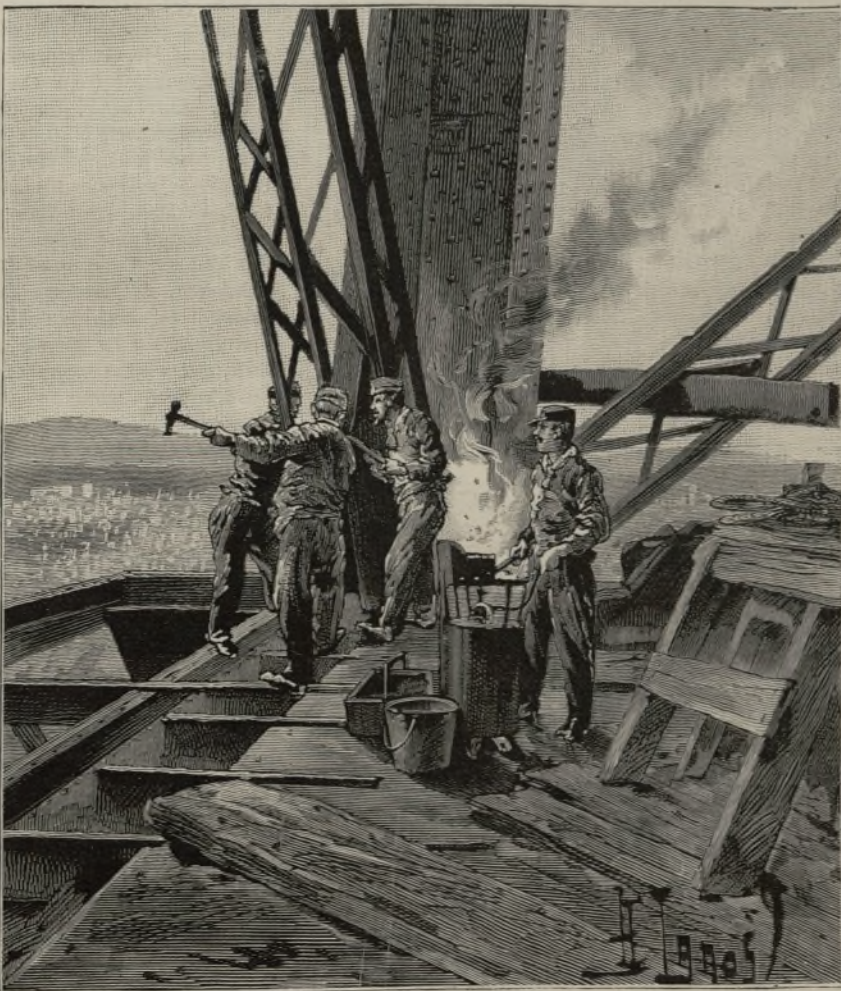
RIVETTING A BOLT
