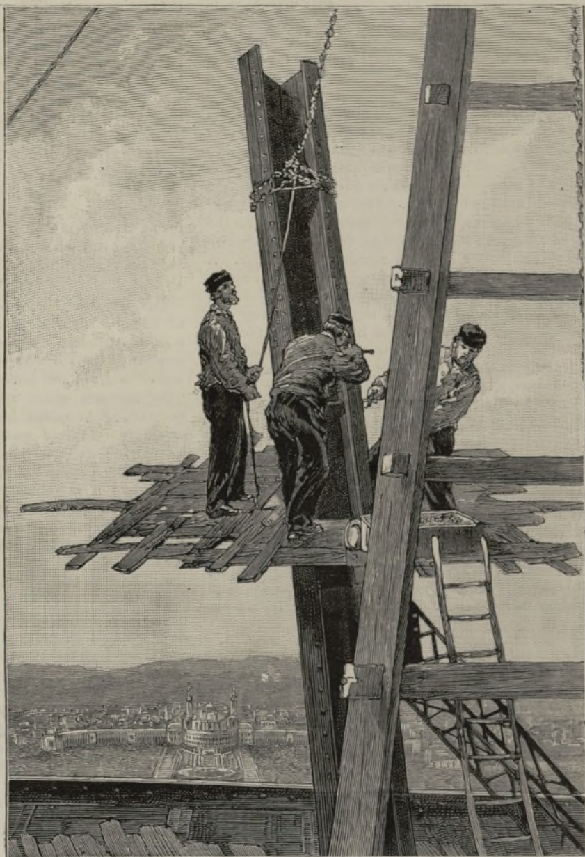
PLACING A GIRDER IN POSITION
