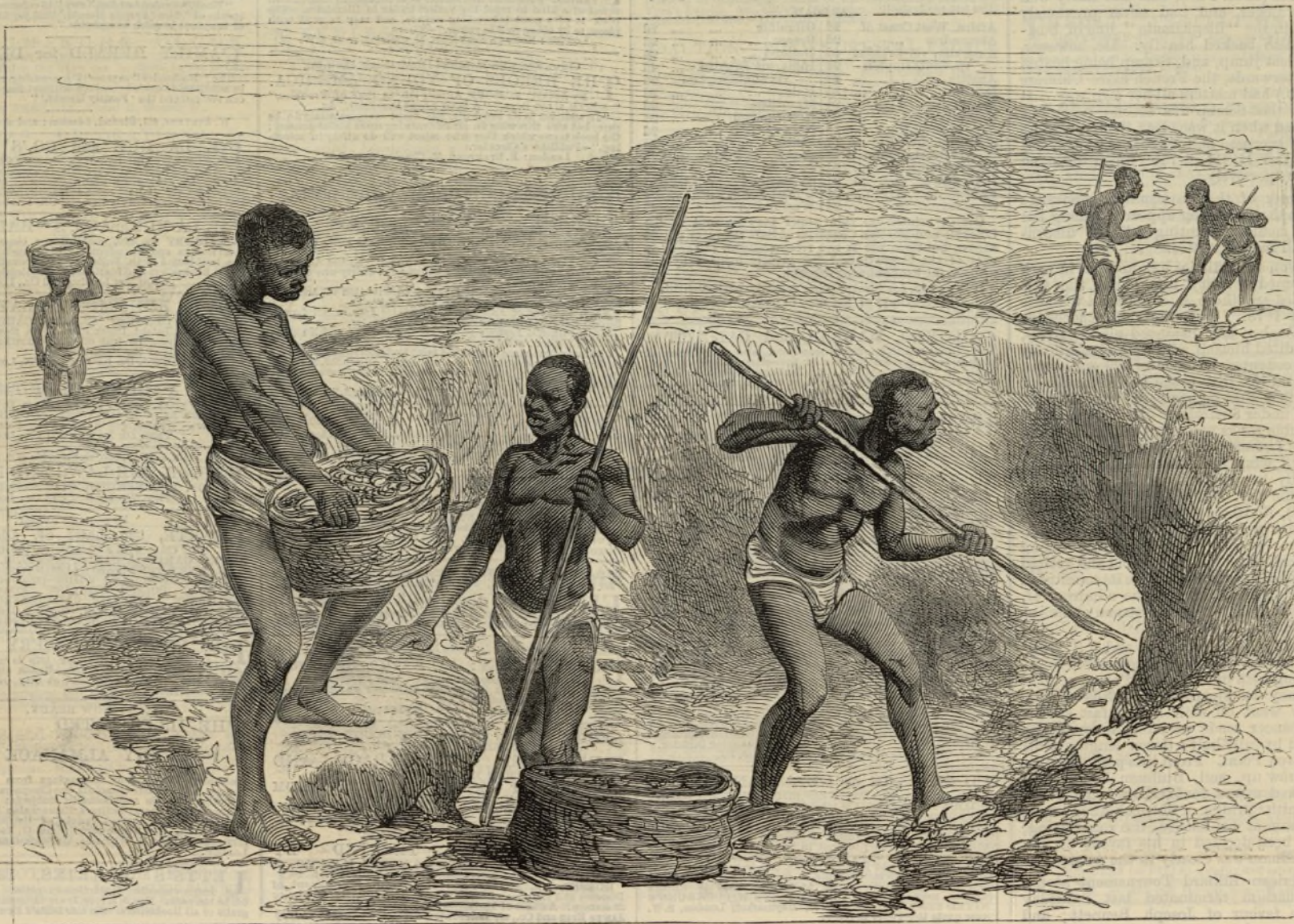
SKETCHES IN AFRICA: BURNING SHELLS FOR LIME.
